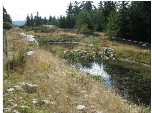
Existing stormwater detention ponds south of Fairwinds Drive
