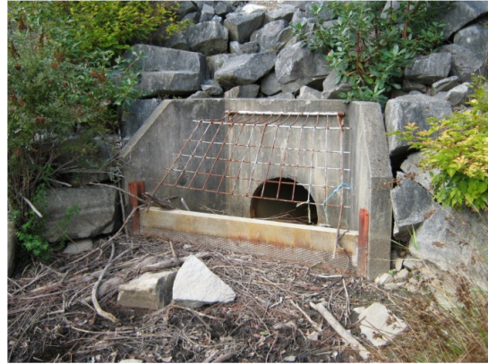
Enos Lake Outlet Structure
