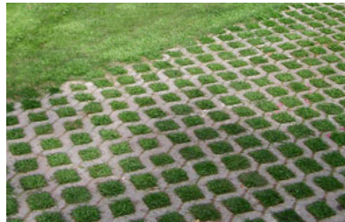
Permeable surfaces, can be used for parking pads to reduce stormwater run-off and maximize infiltration.
