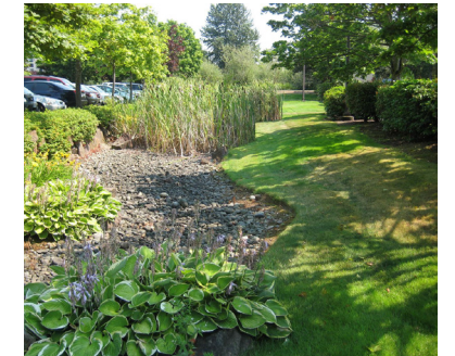
The proposed Project Specific Street Standards allow for stormwater management systems, such as raingardens, within the Right-of-Way.
