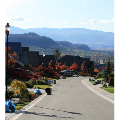
Hillside road design should respond to challenging topography by reducing road platforms and associated cut and fills.
