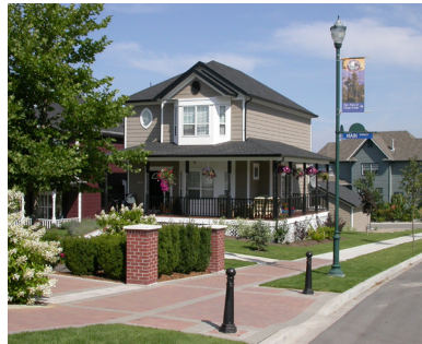
Residential sidewalk using concrete and brick surfacing. Road setback provides a buffer to enhance the pedestrian experience. Utilities are placed within the buffer.
