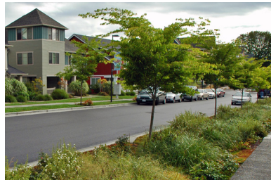
Raingardens adjacent the street absorb and filter stormwater while contributing to the streetscape aesthetic and pedestrian experience.
