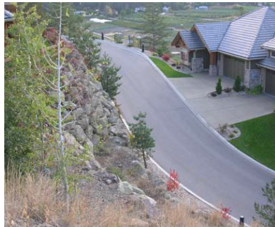
Reduced street Right-of-Ways provide access within fragmented terrain, while minimizing visible cut and fills.
