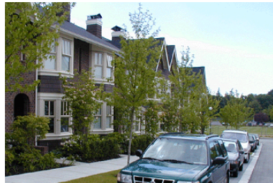
Parking pads adjacent the carriageway are surfaced with permeable materials and linked to raingarden systems.
