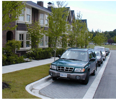
Parking pads provide parking outside the carriageway may be surfaced with permeable material to reduce stormwater run-off.
