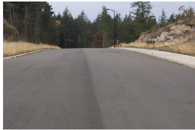
Fairwinds collector roads, shown in the two photos above, swell to 12.7m of paved width and are overscaled for the public realm.
