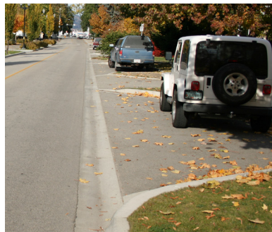
Parking pads adjacent the carriageway reduced the total paved surface.
