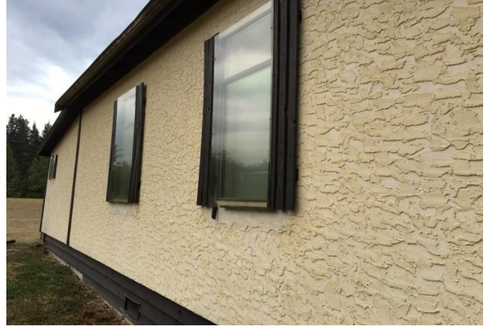
View of side windows
