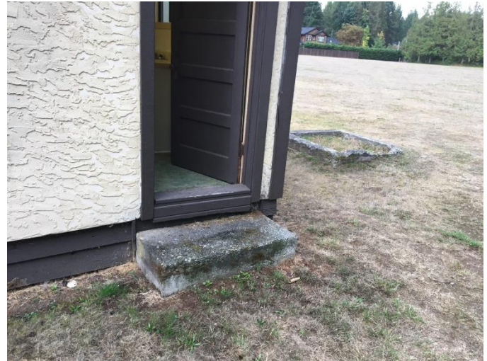
View of rear kitchen door
