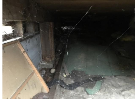
View in crawl space
