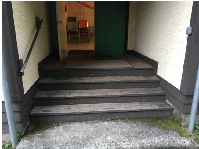
View of main entry door and stair
