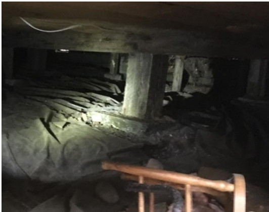
View in crawl space
