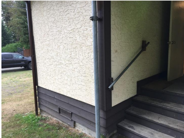
View of handrail at entry stair
