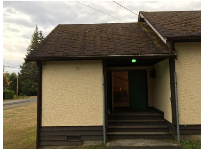
View of roof over entry
