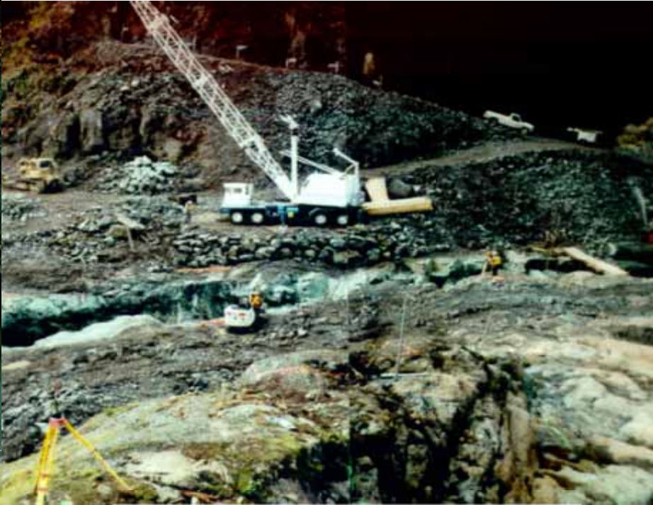
Arrowsmith Lake Dam Construction - 1998
