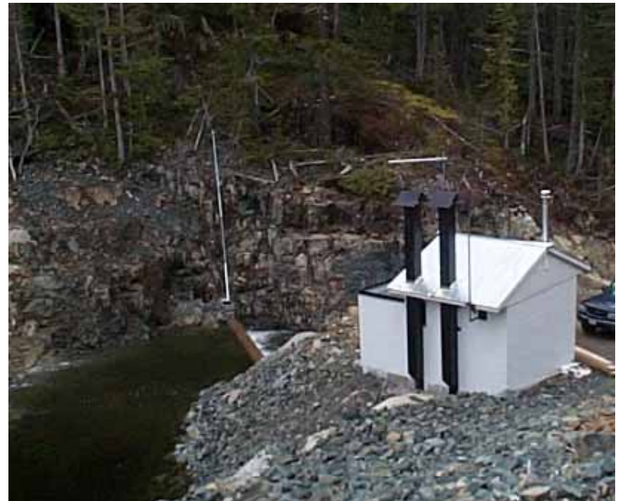
Arrowsmith Dam – Control Station
