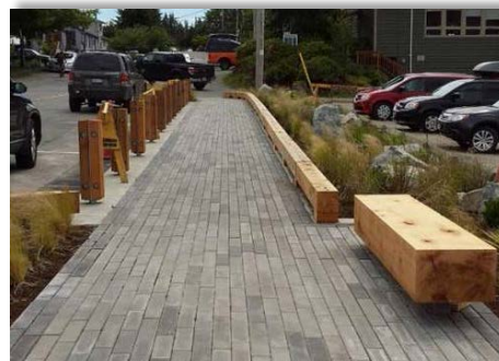
Examples of decorative street furniture with complementary landscaping to define public outdoor spaces.
