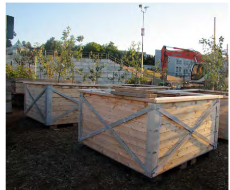
Raised planter boxes on an industrial site in Vancouver, BC. These planters have been designed to be moved by a forklift.
