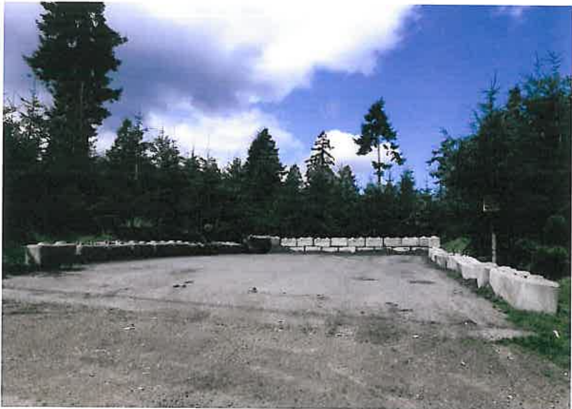
Photo 4. Biosolids containment area (currently empty) consisting of asphalt pad with concrete lock blocks (view looking northwest).
