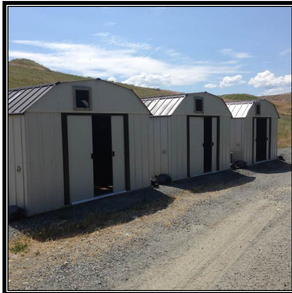
Site aviaries, constructed of metal with transparent panels and screened windows on two sides.
