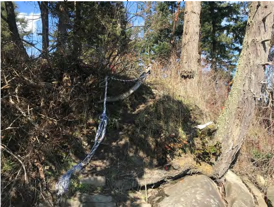
Photo 2: Existing beach access point from footpath.
