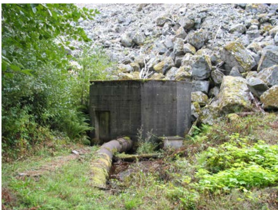
23 - Sluice Valve House
