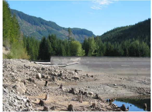
2 - Dam Face North
