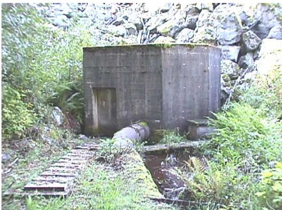
⑤ Dam Sluice Valvehouse
