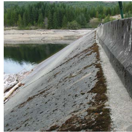
6 – Dam Face – Side View
