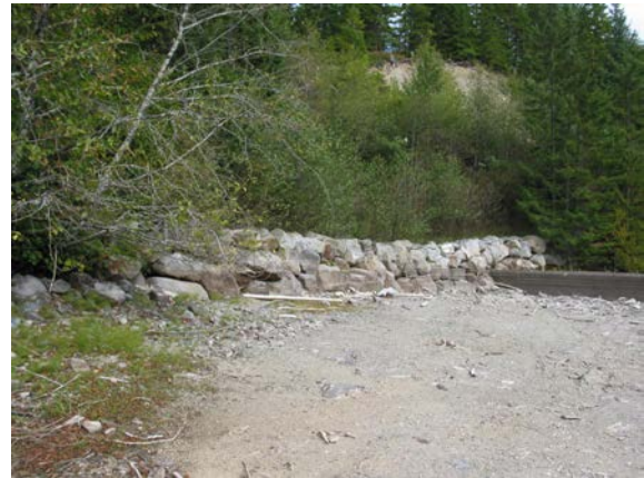
14 - Spillway Abutment RipRap
