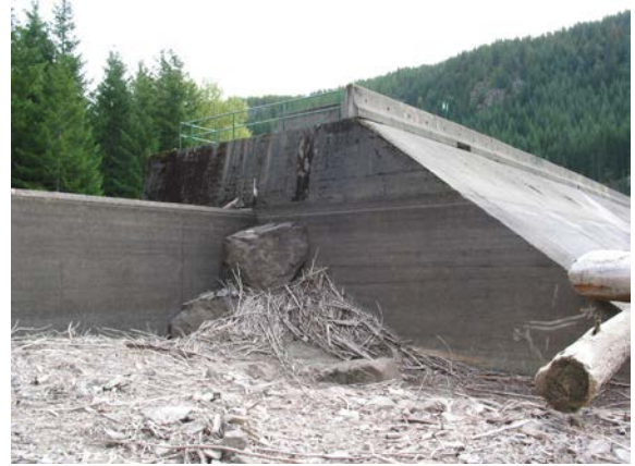
8 - North Dam Abutment
