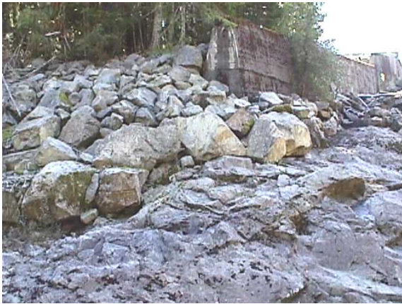
③ Spillway Wingwall and Riprap
