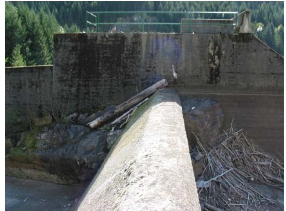
10 – Spillway Dam Crest South
