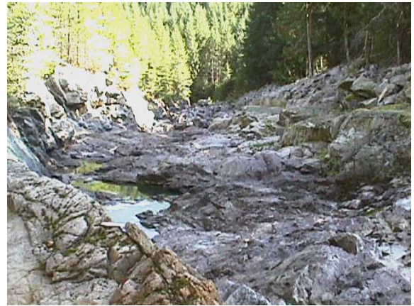
④ Spillway from end of Wingwall to Sadie Creek
