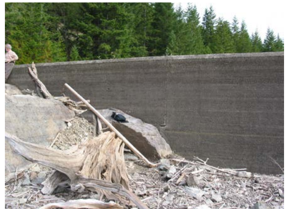
12 - Spillway Control Joint
