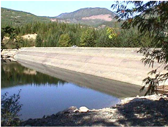
① Upstream Dam Face
