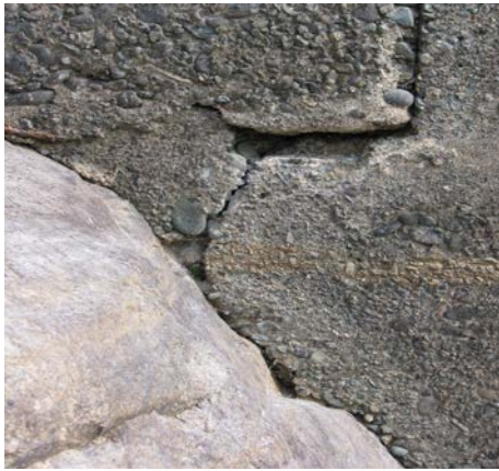
13 - Spillway Control Joint Closeup
