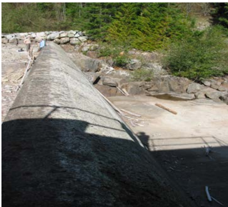
11 – Spillway Dam Crest North
