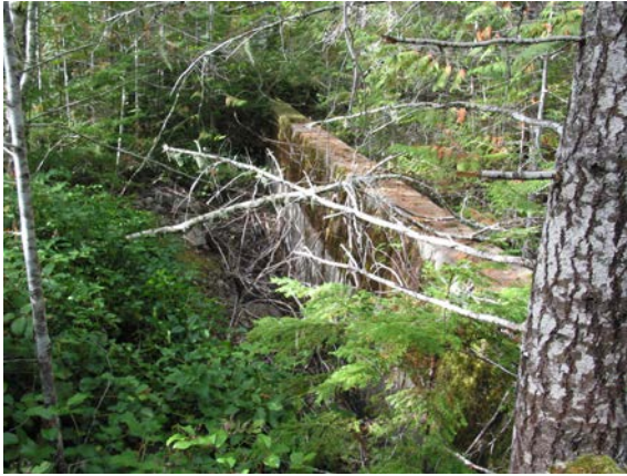
25 - Saddle Dam - Front
