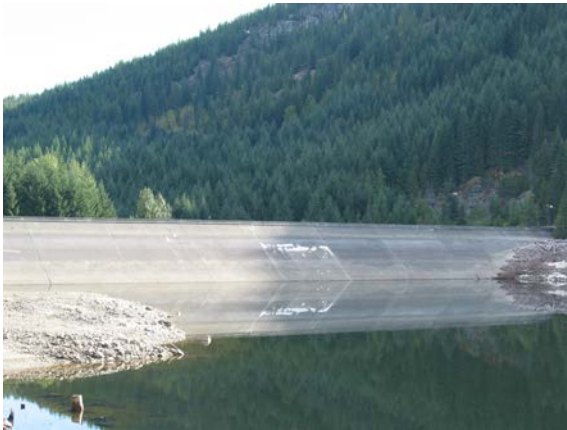
3 - Dam Face South
