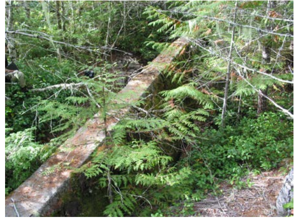
26 - Saddle Dam - Back
