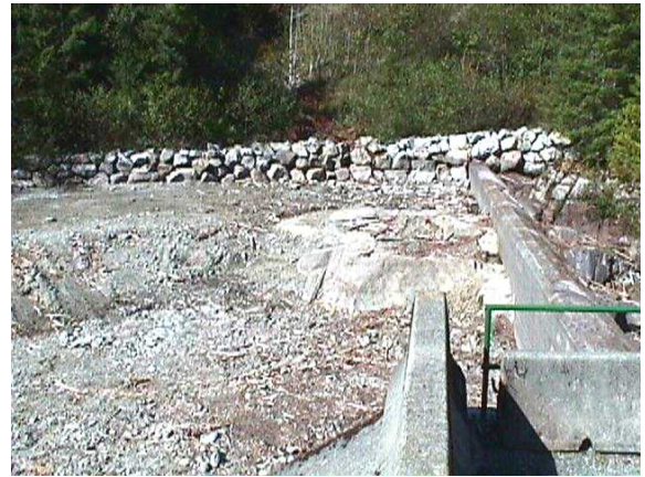
② Spillway Dam
