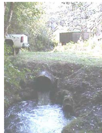
⑥ Sluice and Toe Flows to Sadie Creek
