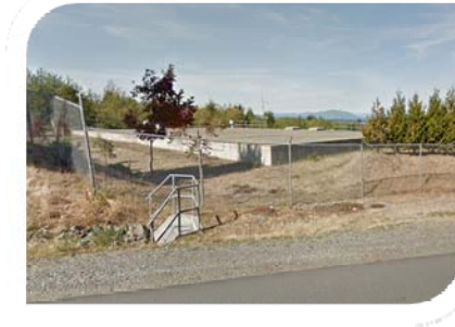
Ware Road Reservoir (2006), 1,887 m 3
