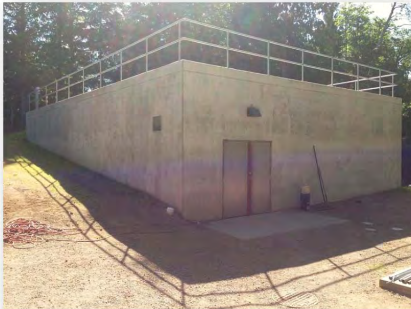
San Pareil Reservoir #2 June 2015
