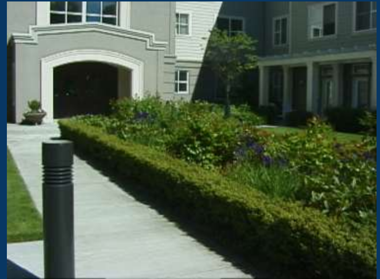
Formal rain garden, Buckman Terrace, Portland, Oregon.
