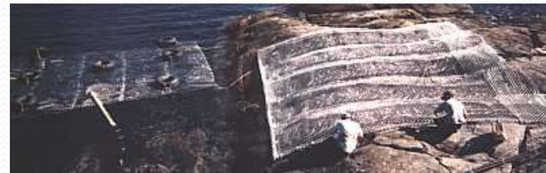
Preparation of heat exchange mats
