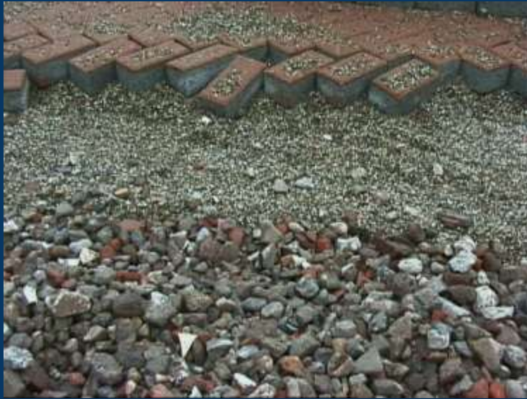
Pervious paving reservoir base.
