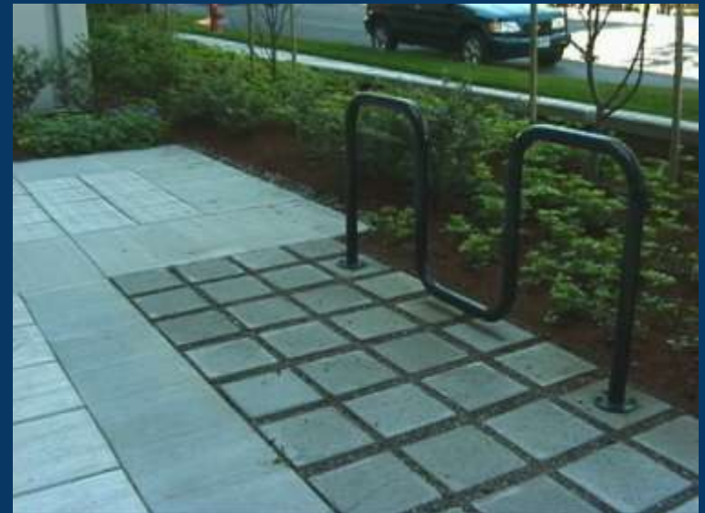
Pervious unit paving with aggregate joints at bike rack.
