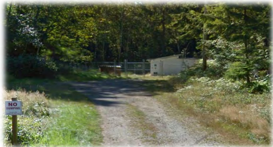
Water Intake Location and Pumphouse
