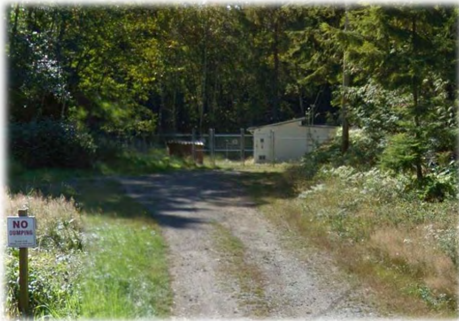
Water Intake Location and Pumphouse
