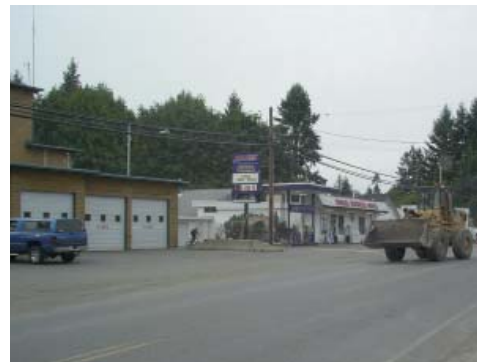
The Cedar village area contains some of the increased density and mixing of land uses sought for the village areas.
