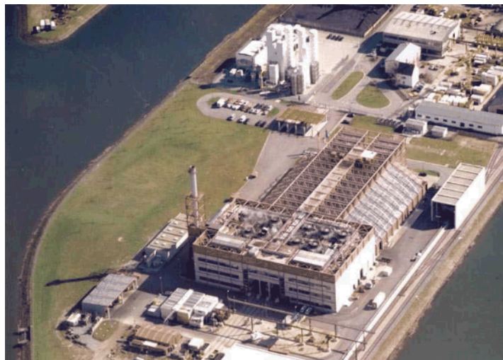
Figure 3-3 Thermosteel high temperature gasification/vitrification facility, Karlsruhe, Germany
