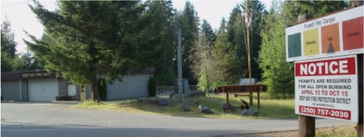
Photo 14. Deep Bay Volunteer Fire Hall.
