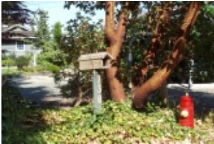
Photo 9. Residential neighbourhoods at Deep Bay are serviced by fire hydrants.
